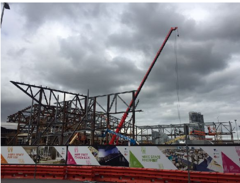
MCEC extension (looking towards north facade) june 2017
