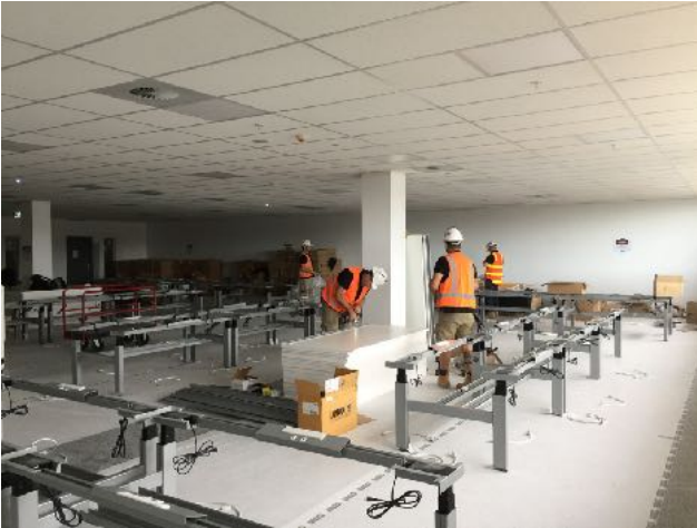
workstations being installed april-may 2018
