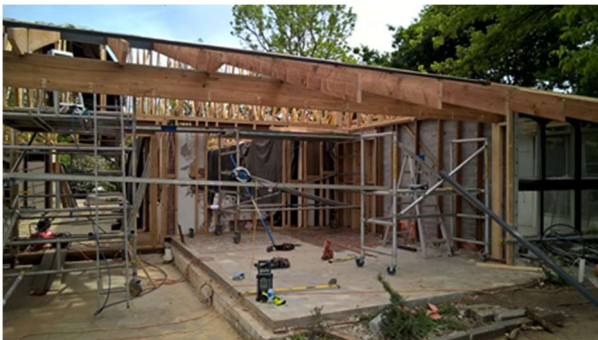
new roof structure to the extended south terrace oct 2015
