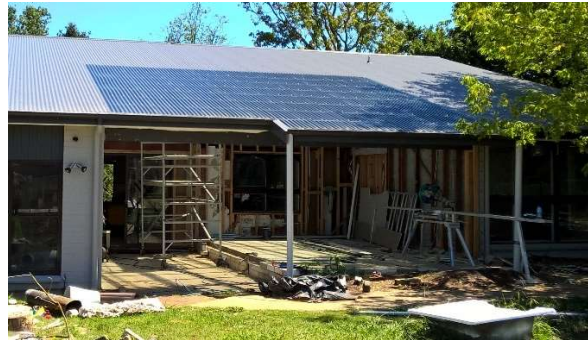
new roof sheeting to the south terrace dec 2015
