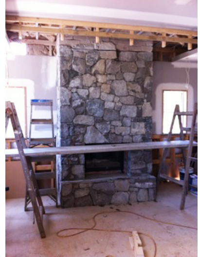
dry stone walling to chimney
