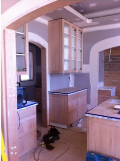
dec 2014 - kitchen cabinetry installed
