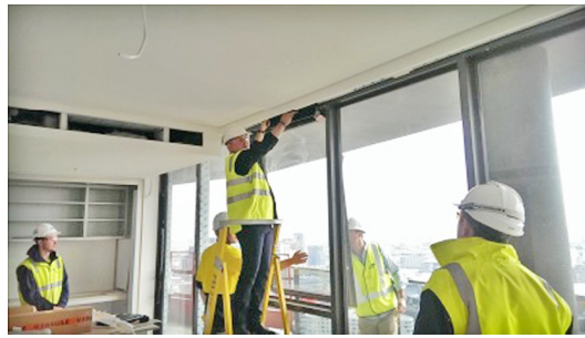
resolving the blind & pelmet detail dec 2014
