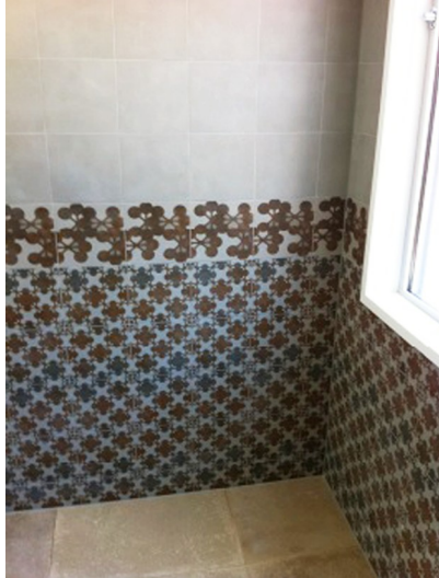
bathroom tiling nearing completion
