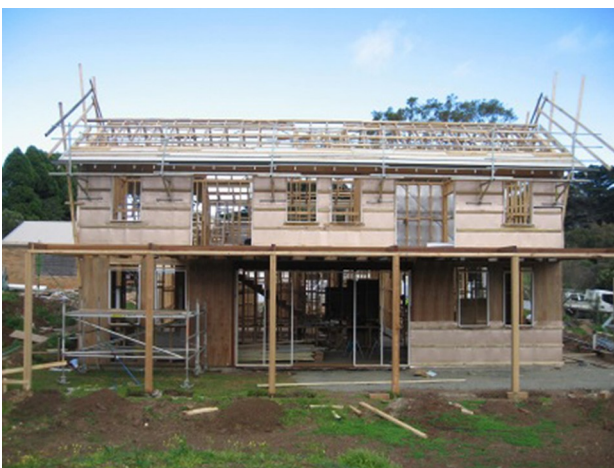
framing almost complete august 2014 (looking south)
